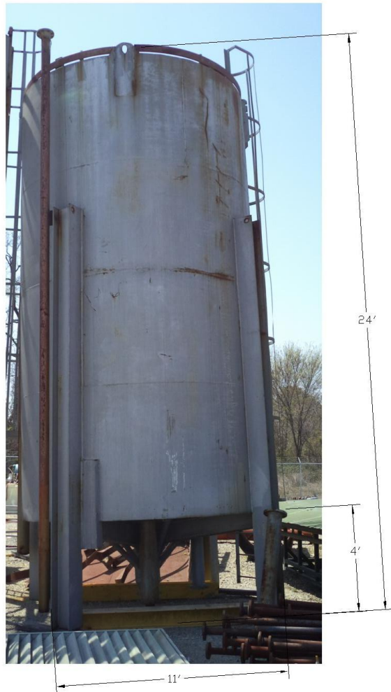
ELEVATION 1-A SILO CAPACITY: APPROX 1900 CU FT
